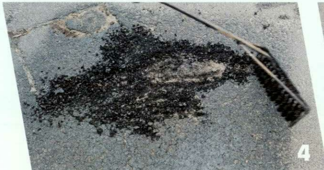
Loose the edges with a rake, remove the dirty asphalt
