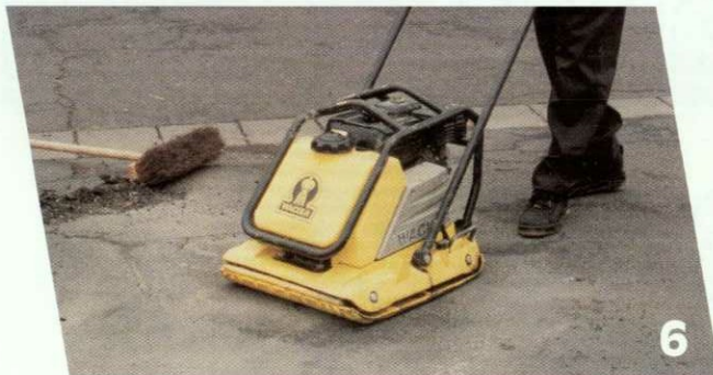
Compact with a vibratory roller or a vibratory plate compactor
