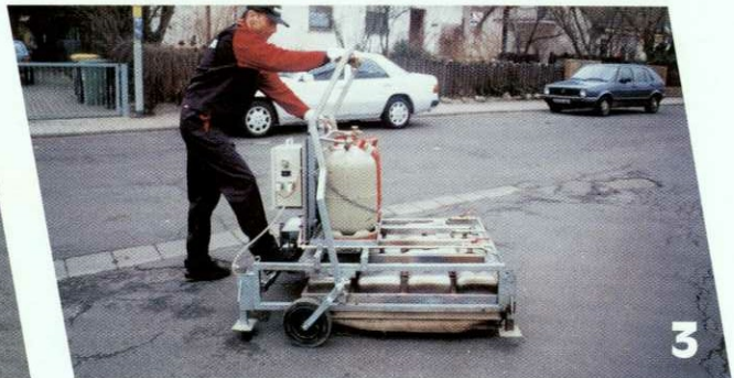
Heat the surface in a controlled manner
