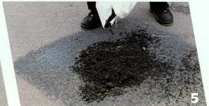
Replace with hot asphalt or C.A.R.-Filling Compound
