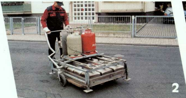
Put the C.A.R. on the surface to be repaired
